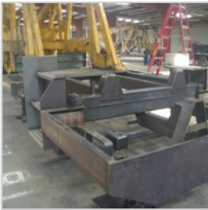
Frame extension in place
